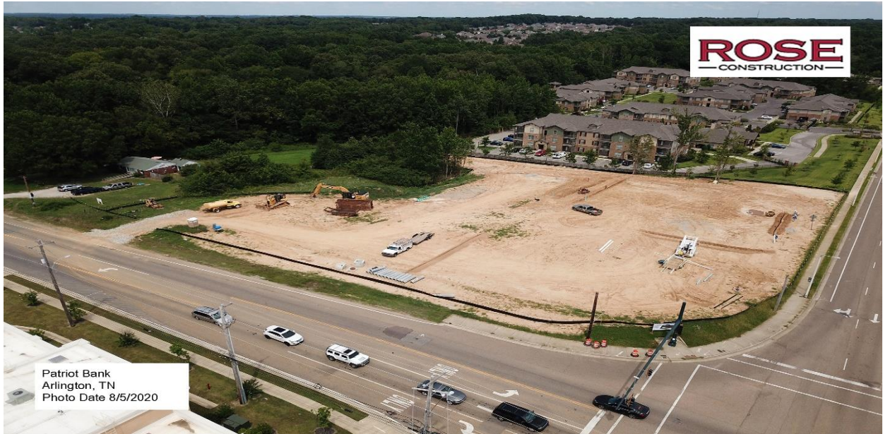
Patriot Bank Jobsite in Arlington, TN
