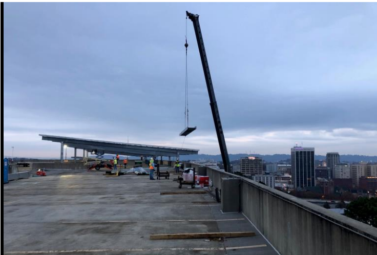
Crews install structural frames for solar panels on the top deck of the parking garage at BlueCross BlueShield Corporate Office in Chattanooga, TN for our client Light Wave Solar.
